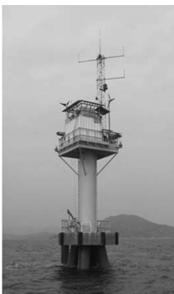
Fig. 5 – Overview of Wind Monitoring Station
