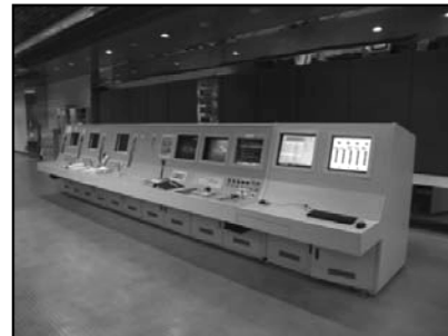
Fig. 9 - Remote Monitoring Computer at Central Control Room
