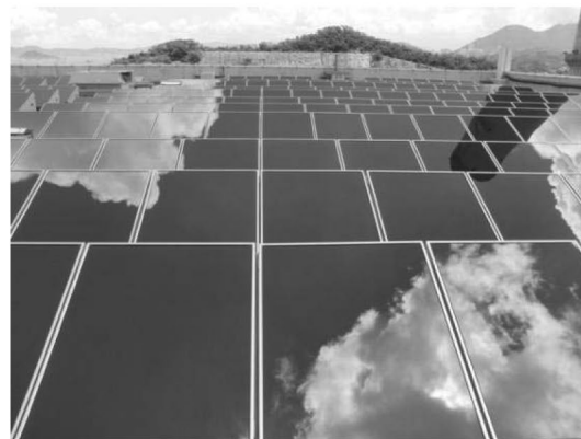
Fig. 7 – Amorphous Silicon Thin Film PV Panel
