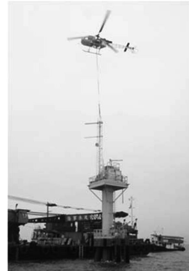
Fig. 4 – Equipment Installation of Wind Monitoring Station
